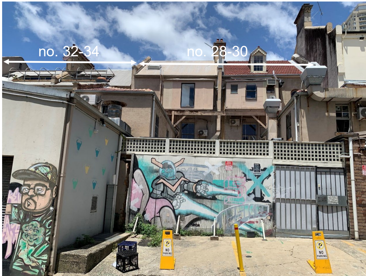
rear of no. 28-34 as viewed from Mansion Lane
