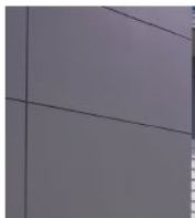
Q - CEMENT SHEET CLADDING WITH BRONZE FINISH
